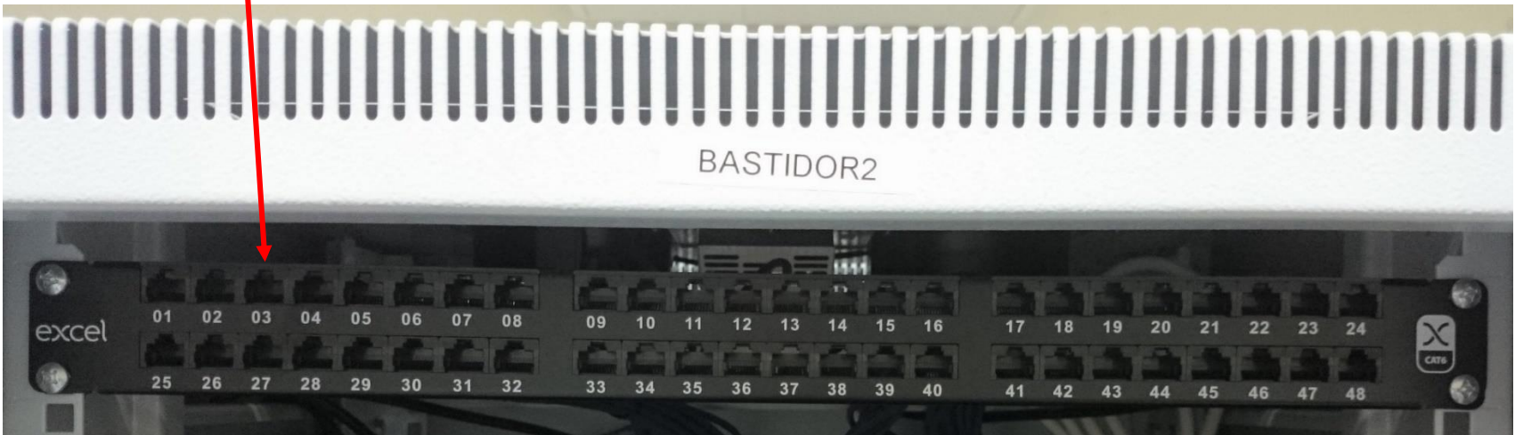
Patch panel no bastidor 2
